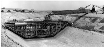
Immediately after World War II, G&Z turns to the design and fabrication of canal construction machinery and supplies its first set of canal machines in 1947. These original machines are used on the Grand Coulee Dam project in Washington State, the Friant-Kern Canal, and the Delta Mendota Canal Project in California. G&Z canal equipment has been used to construct over 80% of the canals in the western United States.
